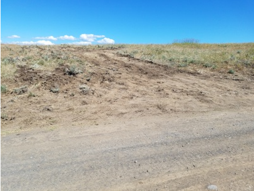
Ruts from road, before
